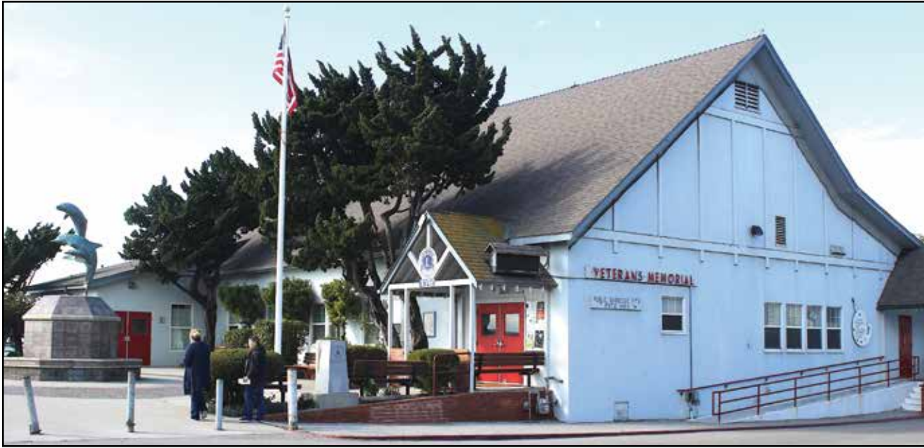
The historic Cayucos Vet's Hall has been closed to the public since May 2016 due to structural problems, but after more than 4 years, there could be good news coming from the County in September. Photo by Neil Farrell
