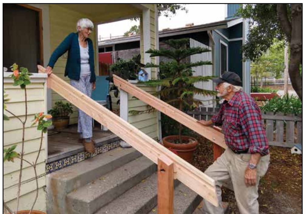
Caption: Volunteer Paul Wolff finishes new ADA Compliant handrails for member Susan Carleton. Photo submitted
