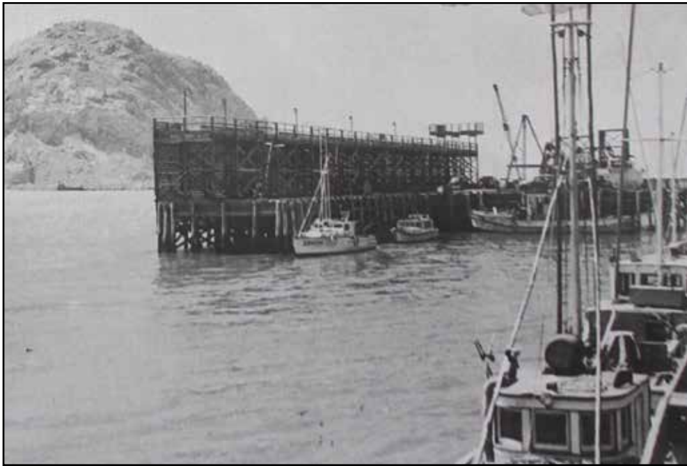
Photo shows the high training walls that were erected on the North T-pier in this photograph taken from about where the South T-pier now stands.
