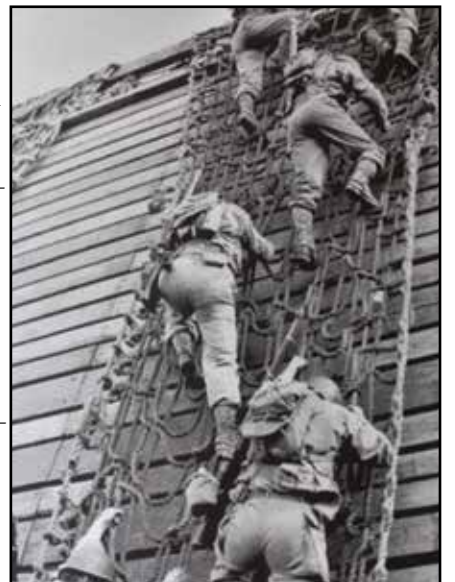
Marines climb cargo nets dangling over the side of a training wall that was constructed on the North T-pier.
