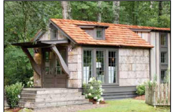
This 'tiny home' (500 square feet) built by Berkshire Hathaway is an example of one type of housing that could go in at Morro Elementary School. Photos courtesy SLCUSD
