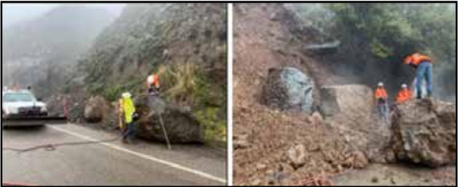
Crews prepare to blast and reduce large rocks near the San Luis Obispo/Monterey County line on Highway 1 on March 11, 2023.
