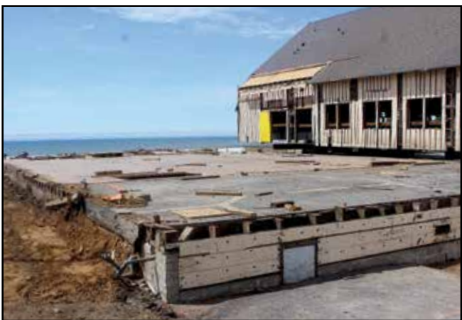
Workers with JG Contracting of Nipomo work on gutting the Cayucos Vet's Hall in preparation for lifting the structure and moving it off the foundation so a new foundation can be poured. Photos by Neil Farrell
