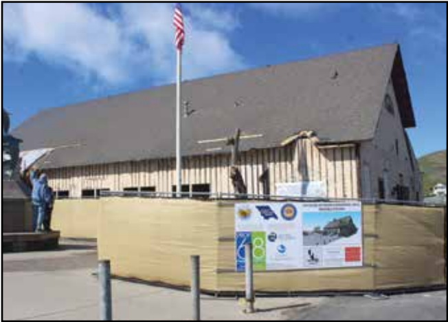
Workers with JG Contracting of Nipomo work on gutting the Cayucos Vet's Hall in preparation for lifting the structure and moving it off the foundation so a new foundation can be poured. Photos by Neil Farrell
