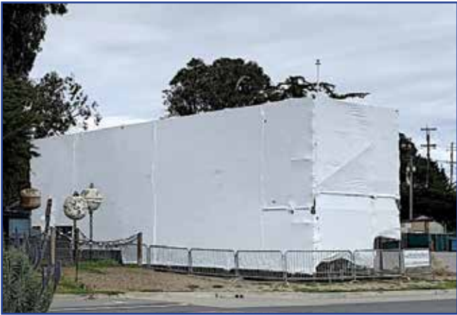
The DSRV Avalon rests behind a 'cocoon' made from shrink-wrap plastic stretched over scaffolding and treated with a propane heat gun, forming a protective shell around the submarine so it can be protected while being painted.
