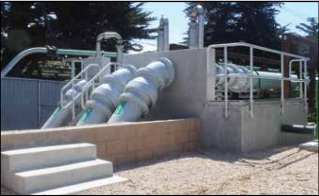
Underground sewer pipes for the City’s WRF Project daylight at Morro Creek and cross in a steel bridge.
