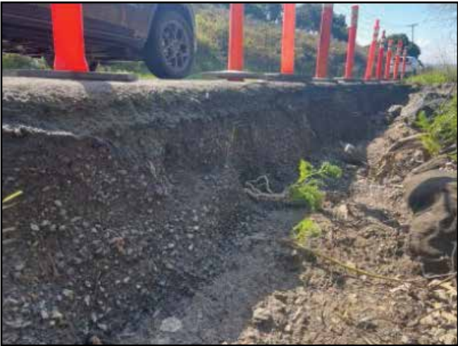
The shoulder on South Bay Boulevard in Morro Bay raised concerns that the asphalt surface would crack off and fall away. Photo submitted
