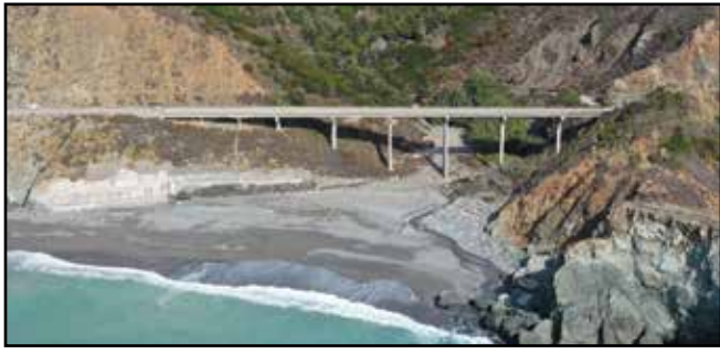
This drone photo shows the Limekiln Creek Bridge on Hwy 1, located just north of Lucia, which is being replaced due to 'chloride intrusion' rusting out the rebar inside the bridge's concrete pillars. Caltrans plans to have a replacement bridge in place by November 2030. Photo courtesy Caltrans
