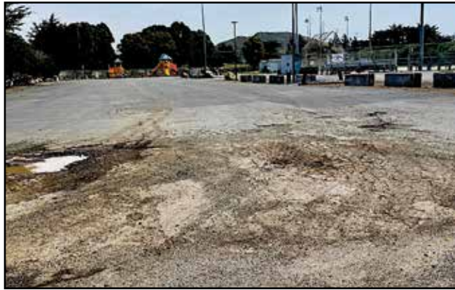
This photo taken by the City of Morro Bay in July 2022, shows a large area of the Lila Keiser Park parking lot that has completely failed. That lot and the police department's annex yard will get repaired and repaved. Photo courtesy City of Morro Bay
