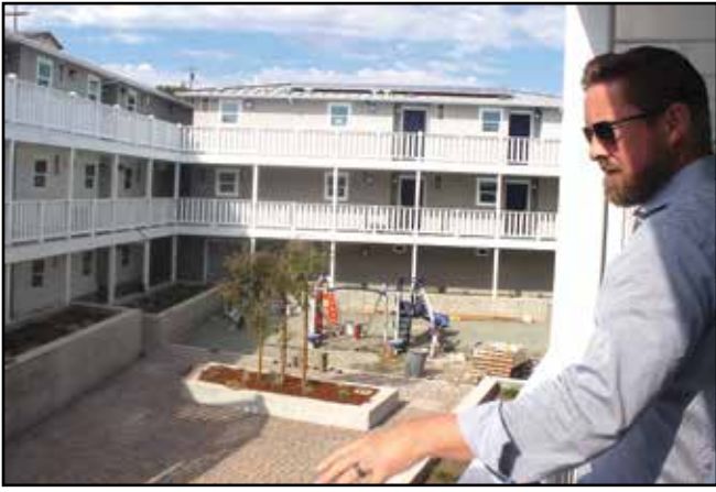
Housing Authority of San Luis Obispo [HASLO] Construction Director, Mike Burke overlooks the interior courtyard of the Rockview at Sunset Apartments in Morro Bay during a tour back in July 2023. Photo by Neil Farrell
