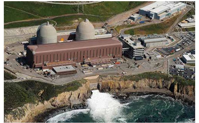
Photo shows Diablo Canyon's twin containment domes, brown power generation building and the ocean outfall discharging heated cooling water into Diablo Cove.
