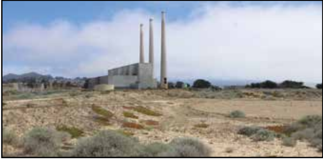
This photo shows a side view of the Morro Bay Power Plant taken from the northern edge of the property, and looking over the top of the site where plant owner, Vistra, hopes to build a battery energy storage facility. The City plans to unveil its Power Plant Master Plan at the Planning Commission's Feb. 20 meeting and the draft EIR for the battery project is expected to be released sometime in the next few weeks. Photo by Neil Farrell
