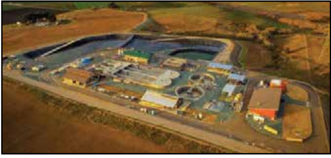
Aerial photo shows the Los Osos Wastewater Treatment Plant shortly after being completed in 2016. File photo
