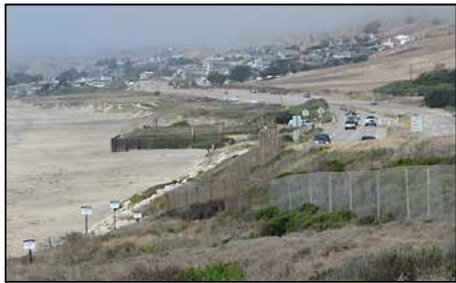
The Morro Bay-Cayucos Connector Bike Way will run from the south end of Studio Drive to North Point in Morro Bay, roughly following the curve of the highway on the ocean side of the fence. File photo
