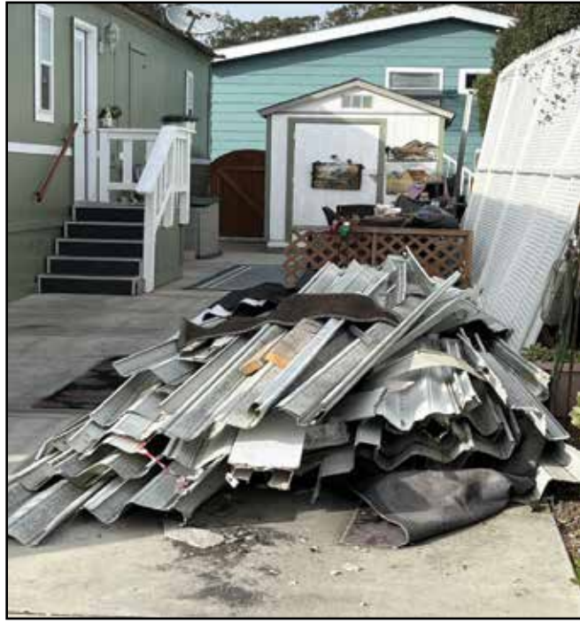
A neighbor removed the remaining structure for safety as storms continued to wreak havoc. Photo submitted
