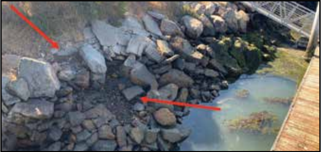
Photo shows where rocks have slipped out of the revetment at the Dunes Street docks, below Anchor Memorial Park.
