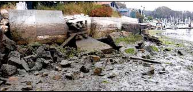
Photo is of the failed seawall by the boat launch ramp that’s been approved for funding of repairs by FEMA.
