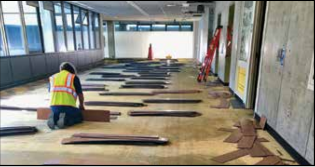
Flooring is carefully pulled from Kennedy Library during its transformation — the first step in giving 10 tons of material a second life through reuse.
