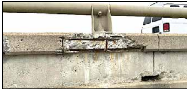
Chunks of concrete have fallen off the southbound Hwy1 bridge over Toro Creek, causing corrosion of the rebar inside. Caltrans plans to replace the bridge starting sometime next spring. Photos courtesy Caltrans
