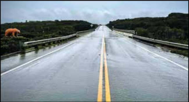
South Bay Blvd. Bridge, heading south. Photo by Paul Irving By Neil Farrell
