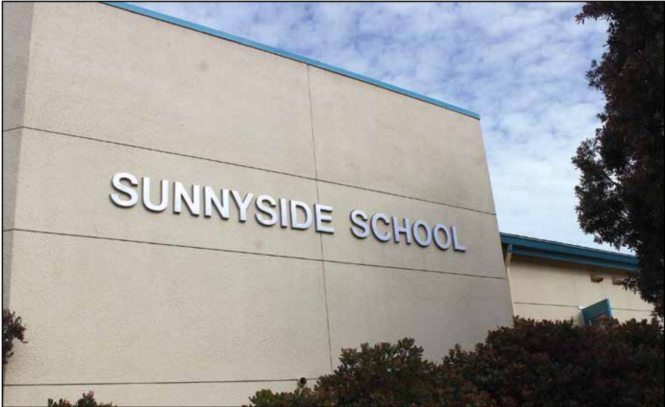
Efforts continue in Los Osos to purchase Sunnyside School from the School District for use by the community. Photo by Neil Farrell
