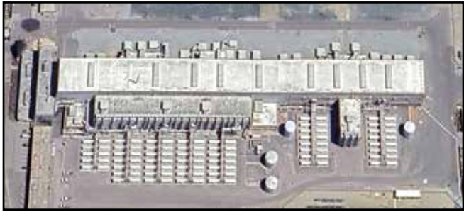
Image shows the 300 megawatt BESS before it burned last January. The EPA has just given Vistra the OK to start removing the destroyed batteries.
