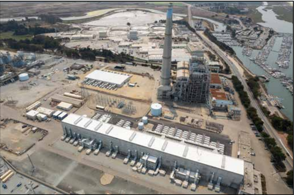
Aerial image from 2022 shows what the Vistra battery plants looked like before the fire. At the right is a glimpse of Moss Landing Harbor; center is the old as00 MW power plant that Vistra is dismantling; and to the left of that is a BESS facility owned by PG&E. Photos courtesy U.S. EPA
