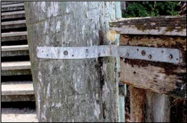
Close-up of strapping that’s been installed to firm up the railing to the wooden piles supporting the stairs.
