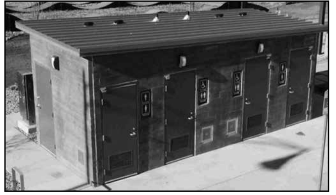
Photo is of the new public restroom the City purchased to install at Coleman Park. Made by CXT, it’s a pre-fab concrete structure that comes ready to install with a crane. The restroom is scheduled to arrive on Memorial Day.
