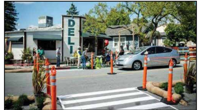
Caution poles designed to slow traffic at a busy pedestrian crossing is one example of a pop-up safety project. SLOCOG is taking applications now for its 2025/2026 mini-grant program. Photo courtesy SLOCOG
