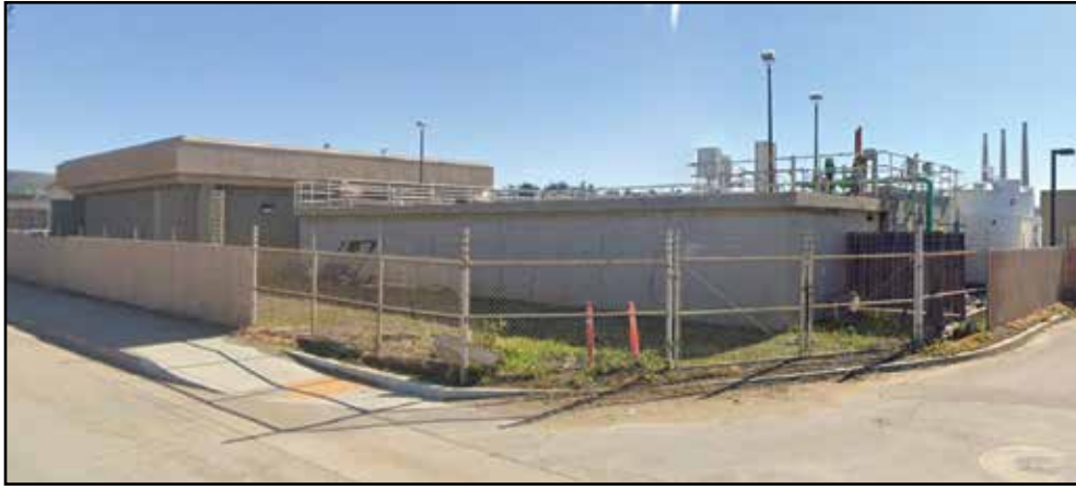
Morro Bay's old treatment plant located on Atascadero road. a good recommendation back to the board."
