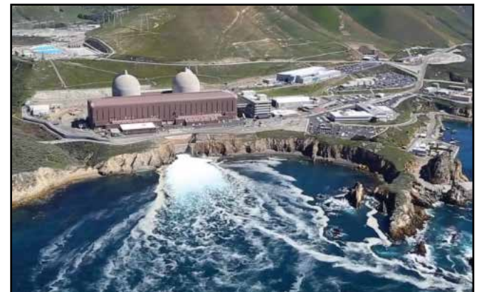
Aerial view of Diablo Canyon with its twin containment domes, brown power building and seawater outfall into Diablo Cove. Submitted photo
