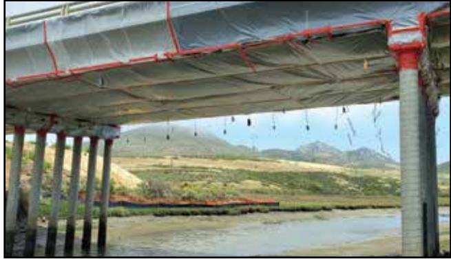
South Bay bridge wrapped to prevent swallow nests. Photo by Dean Thompson
