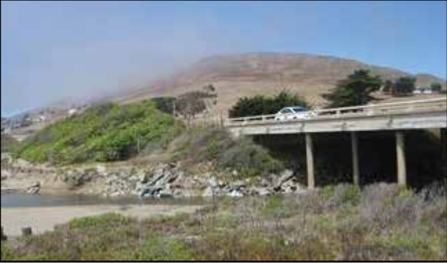
Photo taken from North Point Natural Area in Morro Bay shows the area of Toro Creek that the connector bike path bridge will have to span. Of note, the Hwy 1 bridge shown here is in the process of being replaced by Caltrans. Photo by Neil Farrell
