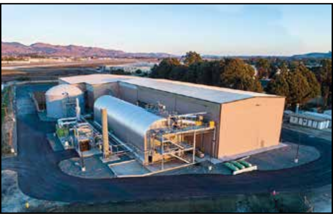
Kanadevia Inova Anaerobic Digester. Photo submitted
