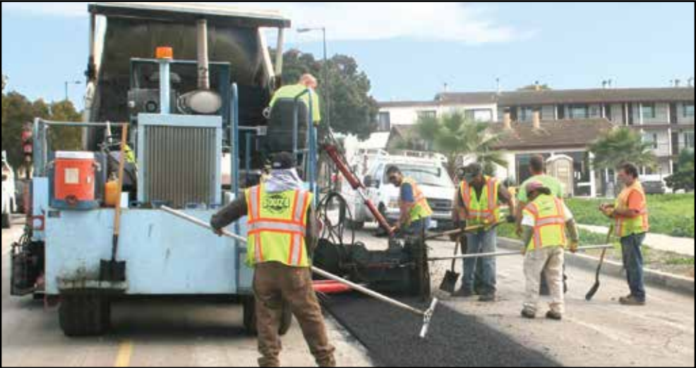
Road workers repair a stretch of Harbor Street in 2015, during the City of Morro Bay’s annual street paving repair job. Photo by Neil Farrell
